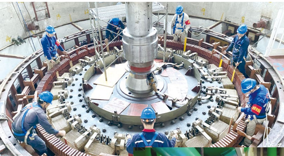
Grade A overhaul site of the No.1 Unit of Datang International Nalan Hydropower Development Company
