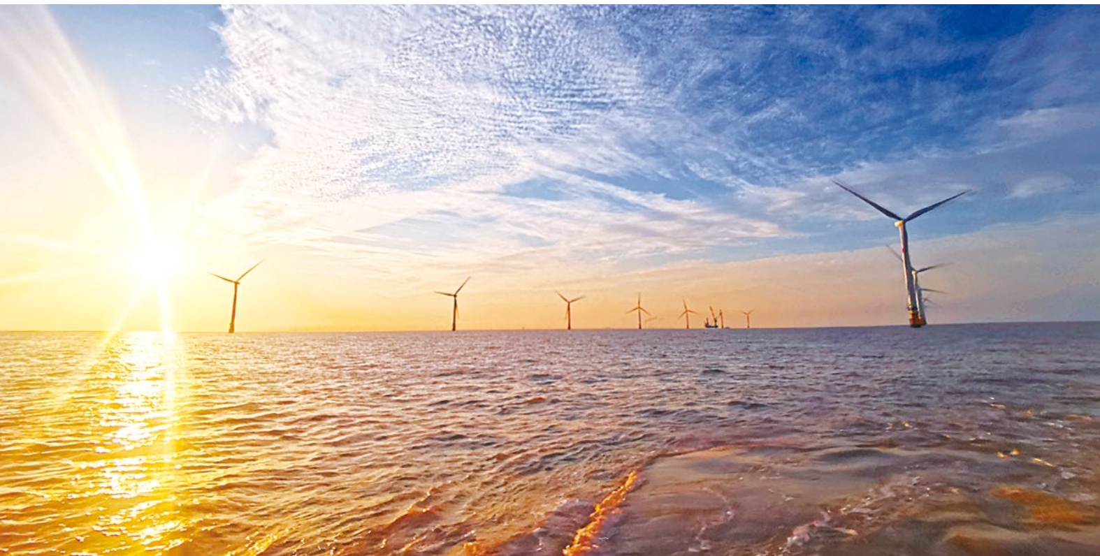
The offshore wind farm of Datang Binhai Offshore Wind Power Generation Co., Ltd.
