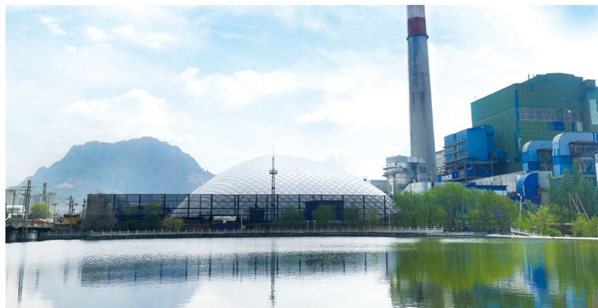
Datang International Xiahuayuan Power Plant has invested RMB 13 million in its closed renovation of coal yard, which covers 14,175 m 2 and stores coal of 45,000 tons, making an outstanding contribution to maintaining air quality during the Beijing 2022 Winter Olympics.
