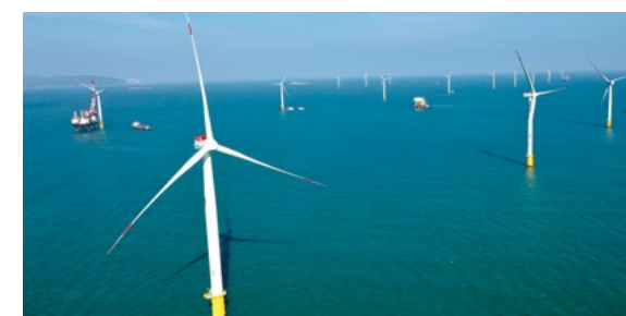
The official launch of Datang Nanao Lemen I Offshore Wind Power Project opens a new chapter in developing offshore wind power in eastern Guangdong
