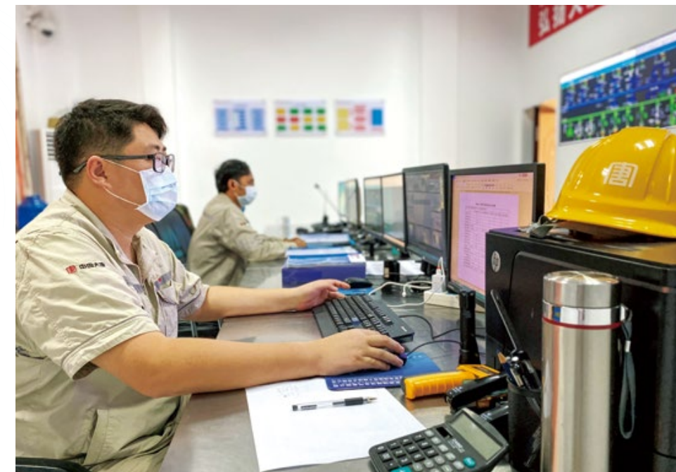
Employees at Pursat Substation of Cambodian Power Grid Co., Ltd. work in front of the monitors.
