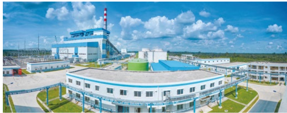
▲ Sumsel Power Plant of Indonesia Datang Sinar Mas Power Co. Ltd.
