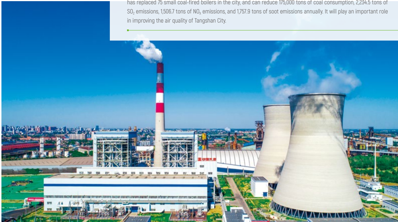
▲ 2 x 350MW ultra-supercritical power and heat generating units of Tangshan Thermal Power Co., Ltd. put into operation.
