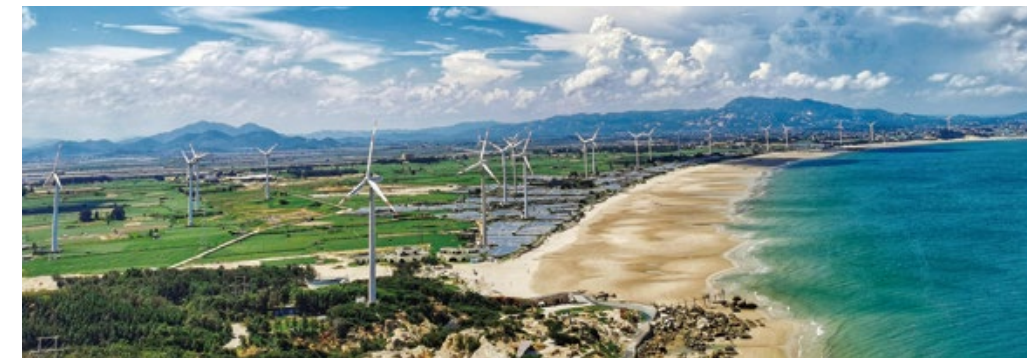
▲ A wind farm under the New Energy Business Division, Fujian Branch of CDT
