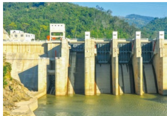
▲ The Taiping River Hydropower Station is the first hydropower project invested and constructed by CDT in Myanmar.
