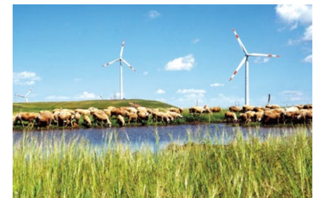
▲ Zhuozi No.1 Wind Farm of the Inner Mongolia Branch of CDT
