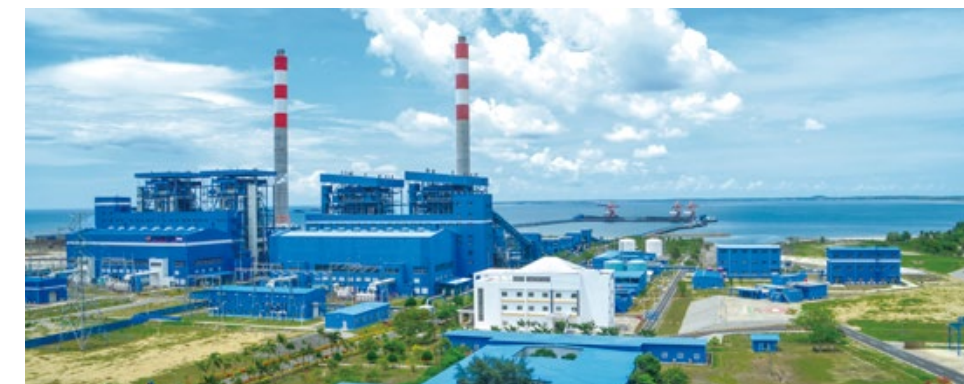
▲ CDT undertakes the operation, maintenance and overhaul of 2x135MW coal-fired units of Jeneponto, Indonesia, which has been highly recognized by Perusahaan Listrik Negara (PLN) and Indonesian proprietors.
